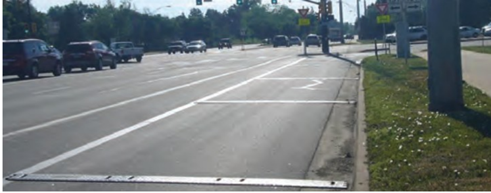
Figure 15. Example of on-pavement sound strips at CRTs [25].
