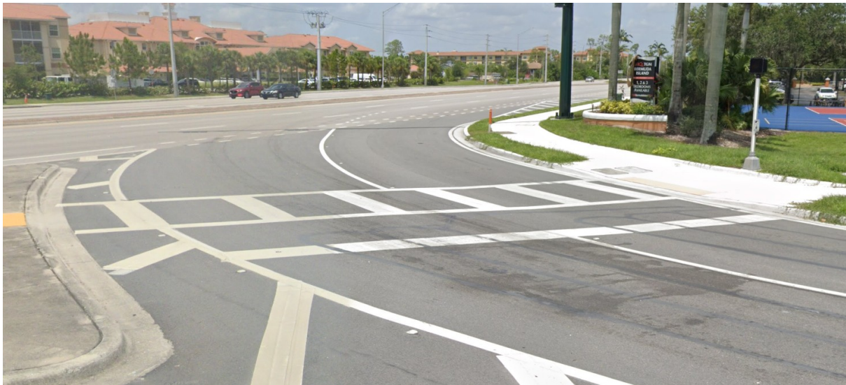
Figure 7. Example of high-visibility crosswalk pavement markings at CRTs [3].
