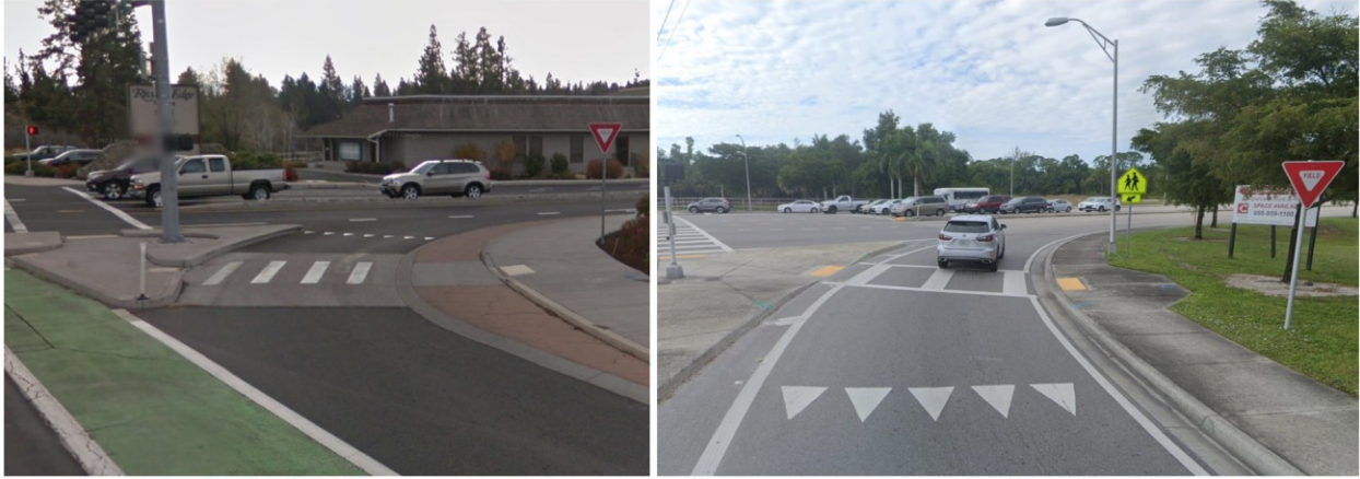
Figure 8. Example of advance yield markings at CRTs [3].
