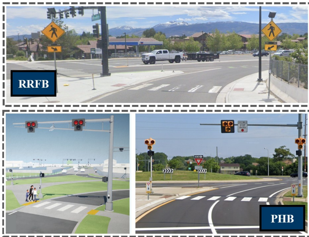
Figure 14. Examples of RRFBs and PHBs used at CRTs or roundabouts [3, 33].
