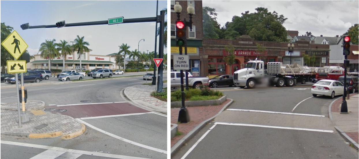
Figure 9. Examples of textured crosswalks at CRTs [3].
